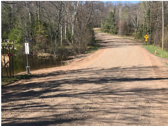
Diamond Lake boat launch May 20, 2020. Grading has been improved from earlier in the year to reduce the slope into the water. It's quite reasonable now but still soft. Pioneer Rd. has been graveled in both directions for about 400 yards as part of the new culvert project, pavement is anticipated sometime in summer 2020.
